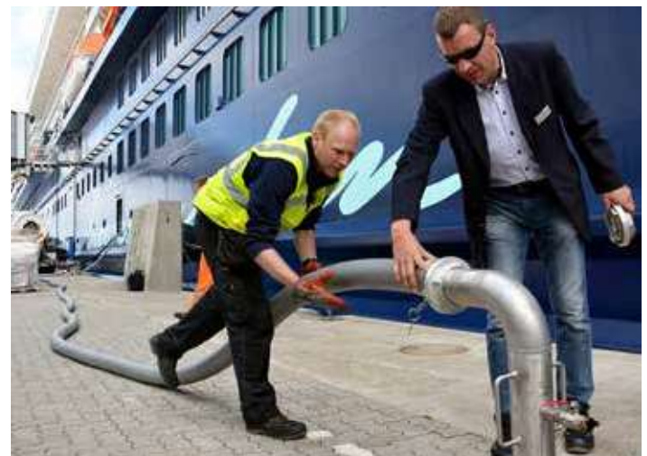
Connecting a sewage waste pipe
